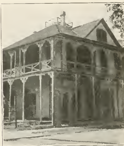
Type of building flat on the ground and with defects in the area wall showing conditions which provide ideal homes for rats.
